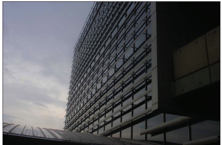
Figure 3. FDA Engineering and Physics Laboratory, facing north.
