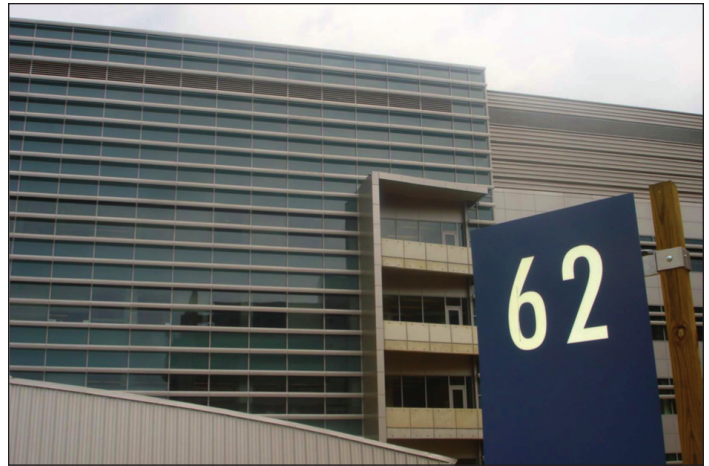
Figure 2. FDA Engineering and Physics Laboratory, facing east.
